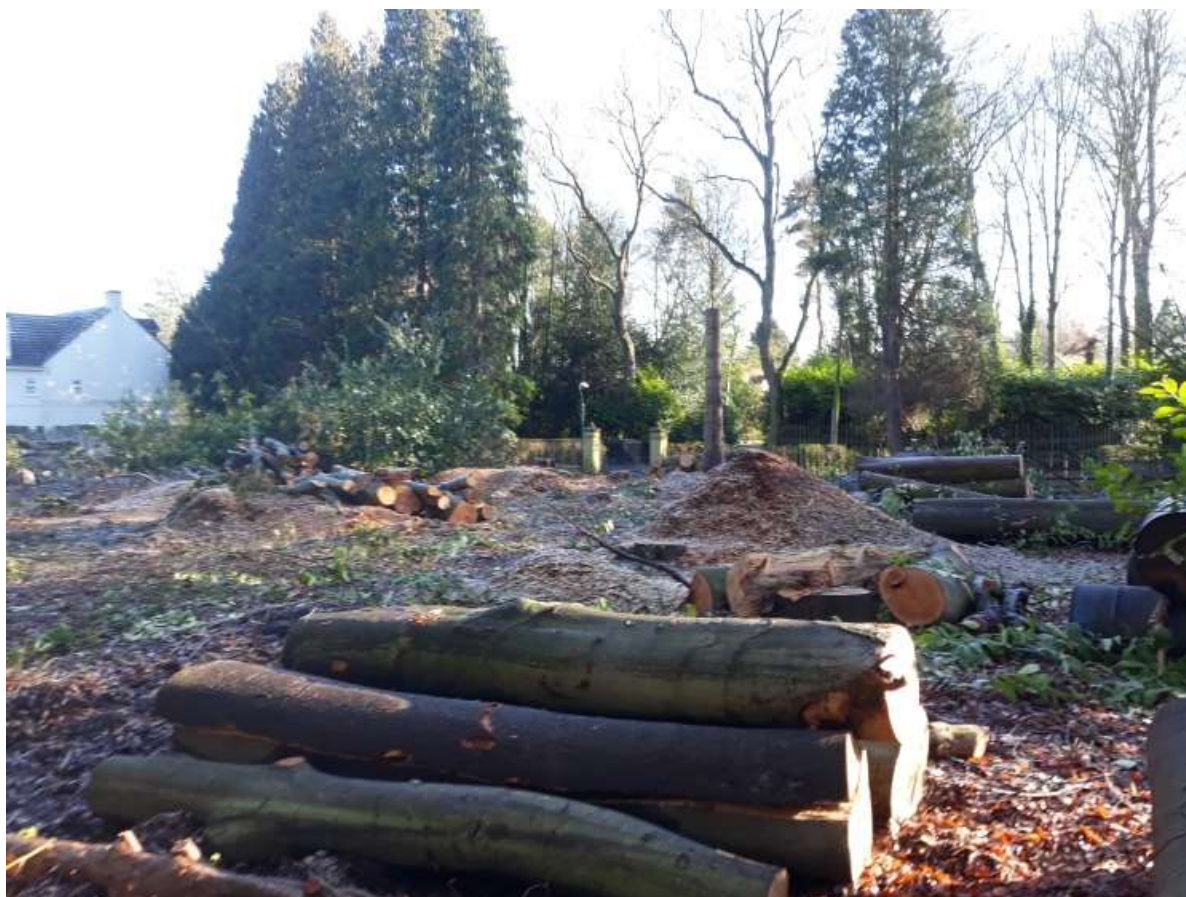
Southern half of the site following clearance
